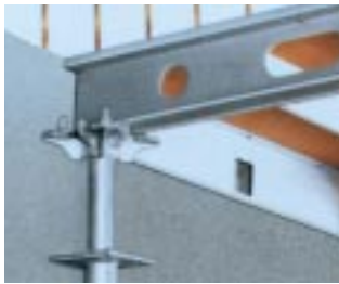
For front-end wall joints the TOPEC bearing is employed.
