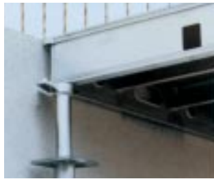
Along the sides of the panels, the edge support provides a tight joint.
